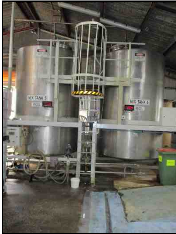
2 X 10,000L DEDICATED SOLVENT MIXING TANKS WITH AUTO SMART FILLER
